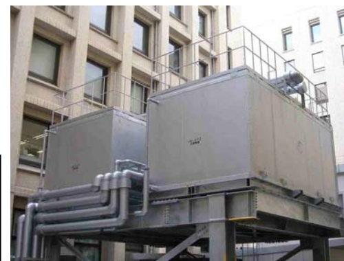
氷蓄熱槽 (1,900kWh × 2槽)
